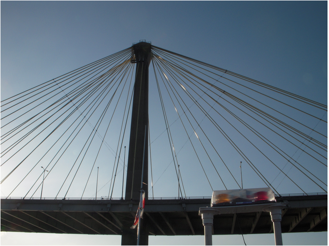
The Clark Highway Bridge carrying Highway 67 over the Mississippi River at Alton Illinois
